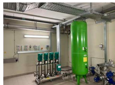
Installation hydrophore
