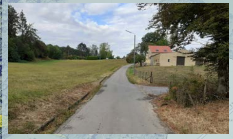
Station de pompage Wolpert
